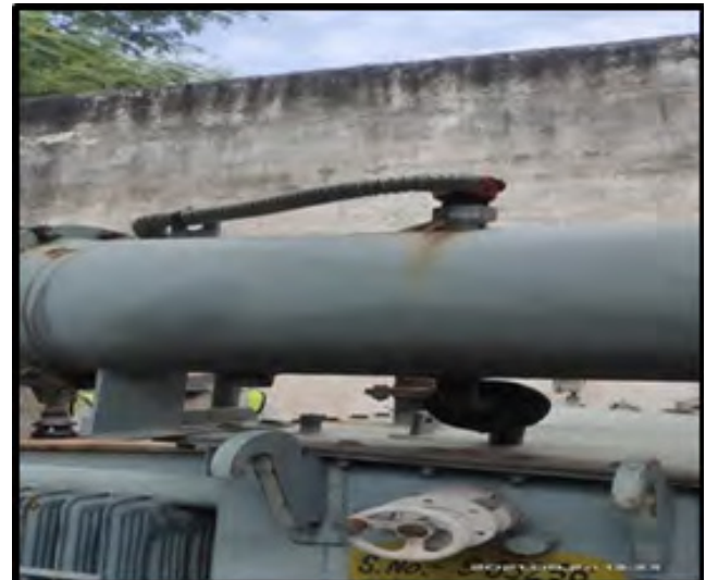
Fig 2: Sensors installed in conservator tank of distribution transformer
