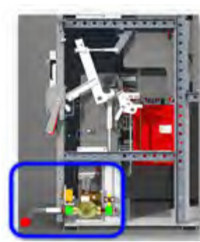
Innovative Maintenance Grounding Device in Motor Control Center with Integrated Interlock
